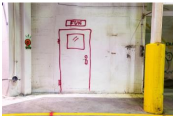
A spray painting remains in an unfinished section of Harbor Island Studios in Seattle, March 11, 2022. (Lindsey Wasson for Crosscut)
